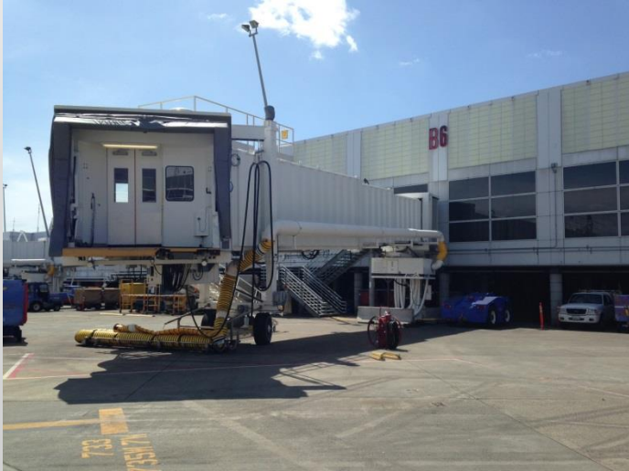
Passenger Loading Bridge at B6
